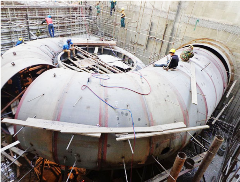
Nam Khan 2 intake structure below.
